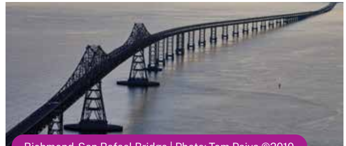
Richmond-San Rafael Bridge | Photo: Tom Paiva ©2010
